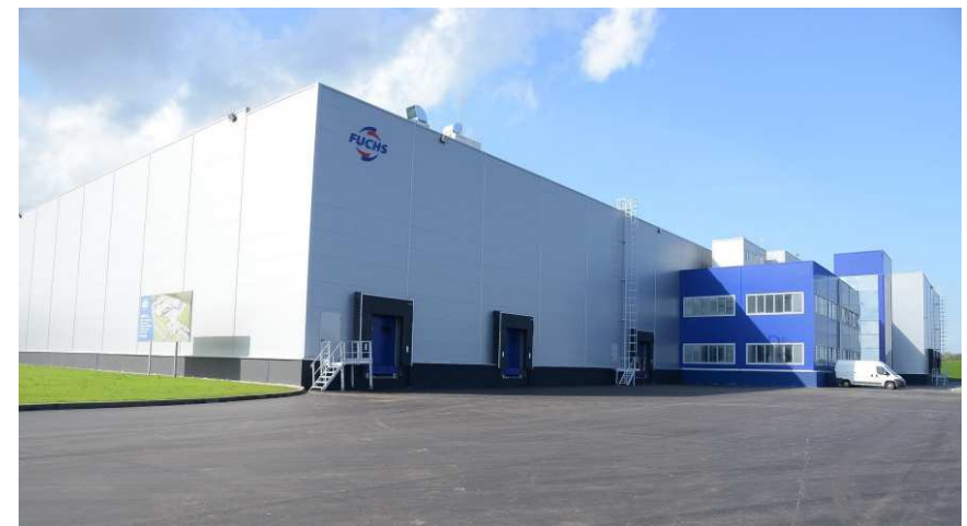
New plant in Kaluga, Russland
