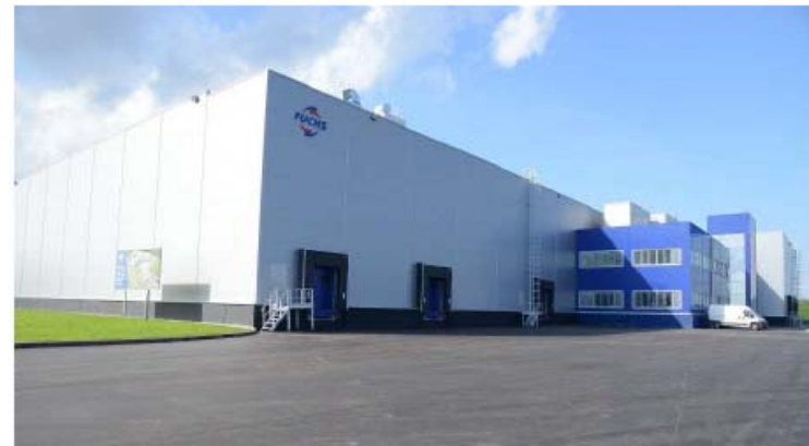
New plant in Kaluga, Russland
