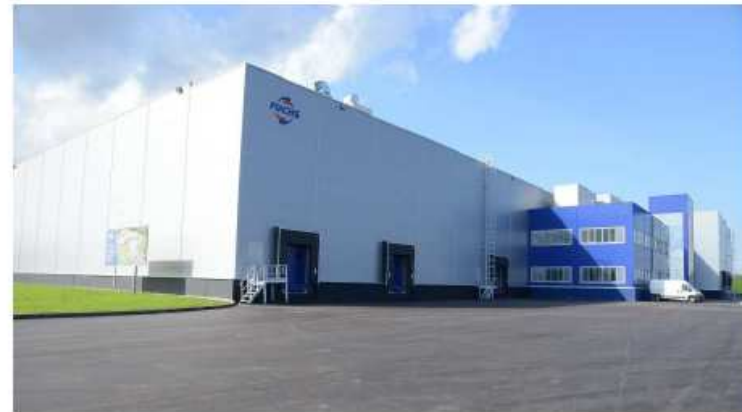
New plant in Kaluga, Russland
