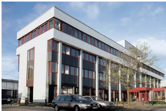
Modernisation of holding building
