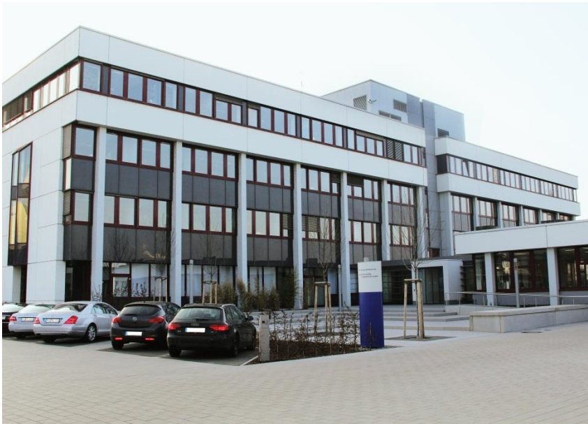
Modernisation of holding building
