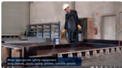
Application of concrete release agents
