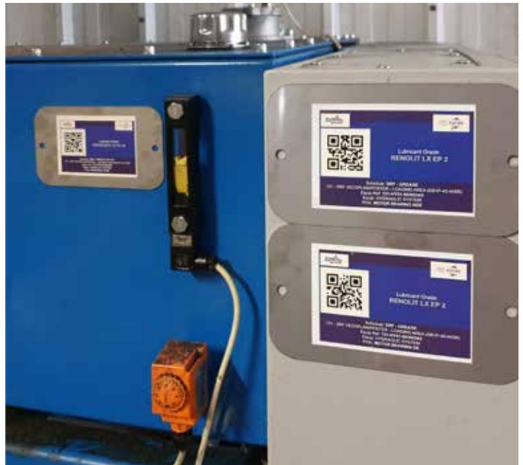
FluidsConnect uses QR code scanners to record machine specific content.
